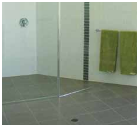
Example of an accessible shower with level entry
