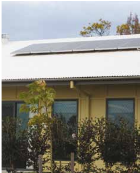
Solar power systems can be identified by a collection of solar panels on the roof
